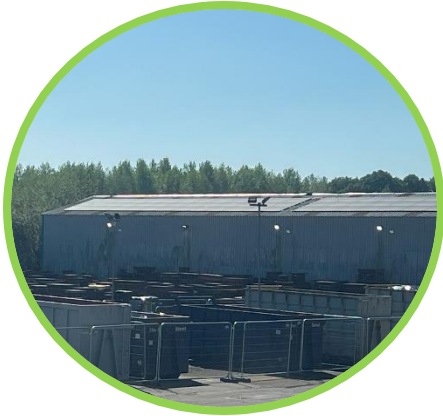
SHS-Scrap Control Area Industrialization
